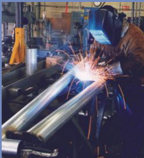
Fabrication of steel truss to support an industrial cover.
