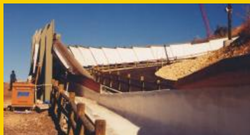
Custom made 12' wide overlapping retractable shades installed at the Utah Winter Sports Park Bobsled Track. Includes industrial spring-loaded top roller and vinyl coated fabric panels.
