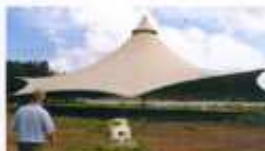
Exhibition hall - 1982 Port-Gentil, Gabon - Précontraint® 1302 Tensile resistance after 18 years: Warp 86% - Weft 76%
