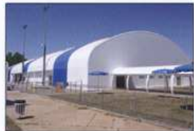
Canberra swimming pool - Australia Removal of membrane installed in 1988 Fabric re-installation in 2009. Recycling in 2010.
