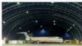
Airbus hangar - 1982 Germany - Précontraint® 1302 Tensile resistance after 22 years: Warp 97% - Weft 84%
