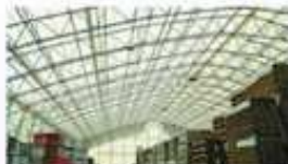
Warehouse - 1989 France - Précontraint® 832 Tensile resistance after 20 years: Warp 91% - Weft 86%
